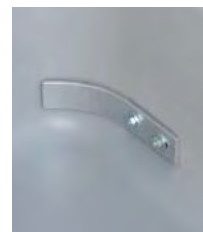
Platform fastening (reinforcement)
